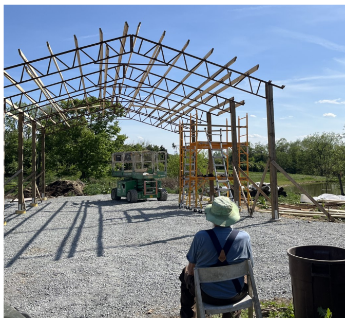
Dale Bahr supervises the construction of the new pole barn at Bahr Farm. This photo was taken roughly 10 days before the project was completed.
