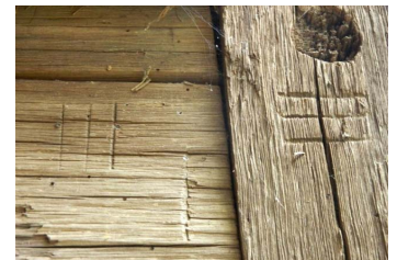
LEFT: Drilling core samples from beams. ABOVE: Finding “marriage marks” etched into the lumber.
